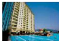
Location, Turkey Project, Hotel
