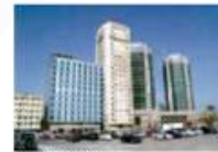
Location, Qatar Project, Office Building
