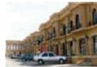
Location, Saudi Arabia Project, Medical Clinic
