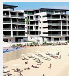
Location: Kenya (Mombasa) Project: English Point Marina
