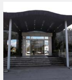
Location: Slovenia Project: Utility company
