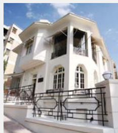
Location: Greece Project: Restaurant
