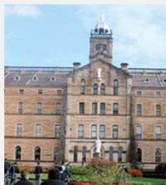
Location: Australia (Sydney) Project: St. Joseph School
