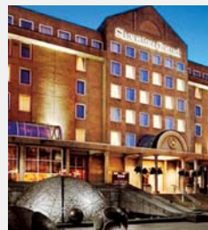
Location: UK (Edinburgh) Project: Sheraton Hotel
