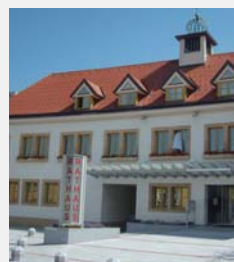
Location: Austria Project: City Hall Traiskirchen
